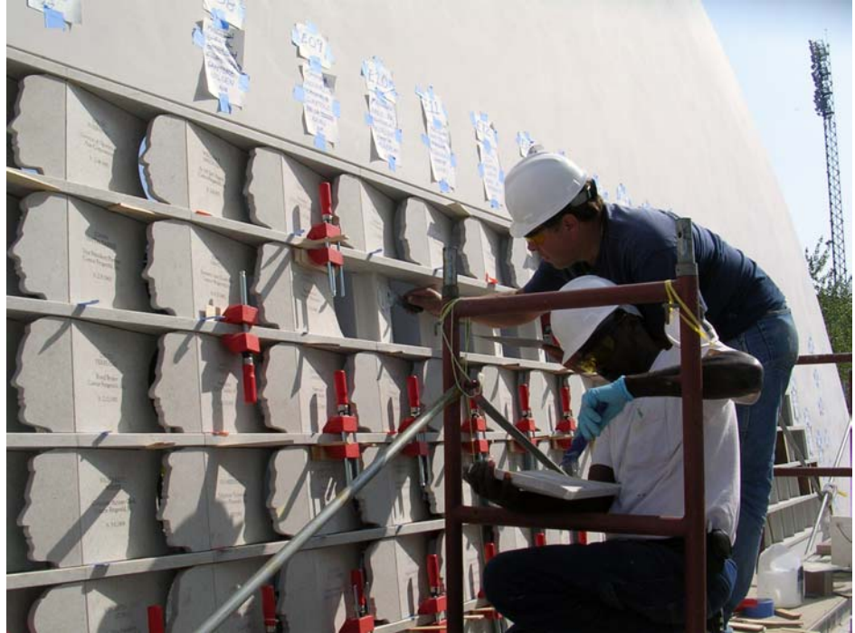
Installation of profile tiles
